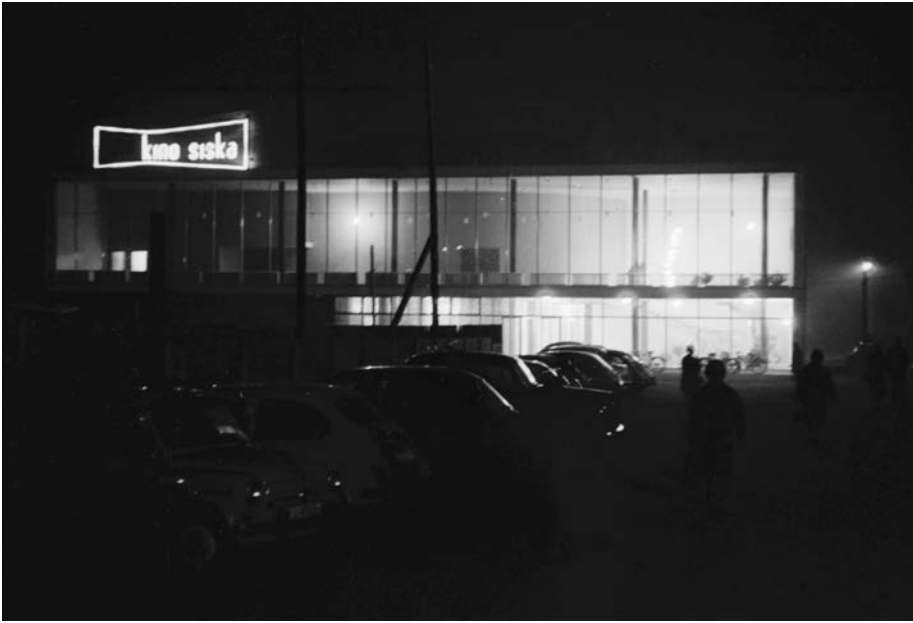
Main façade of Kino Šiška, overlooking the shopping mall on Celovška Street, 1962
